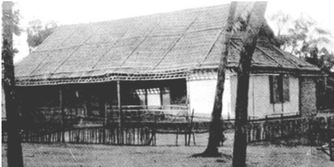
Figure 5- 2 This chalet of the Chemin de fer in Bana in 1924 shows woven mat roofing, walls of mud daub and the floor set on low timber posts. (Sallet, 1924:374)
